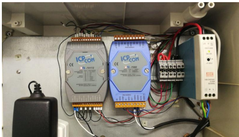
Figure 9.4: Example of ICP CON units used to convert analog to digital signals.
