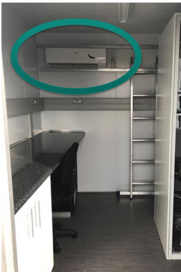
Figure 1.8: Air-conditioner is used to control and maintain the internal temperature of the station.
