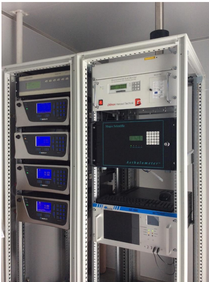
Figure 1.5: Instrument rack used to install monitoring instrumentation.
